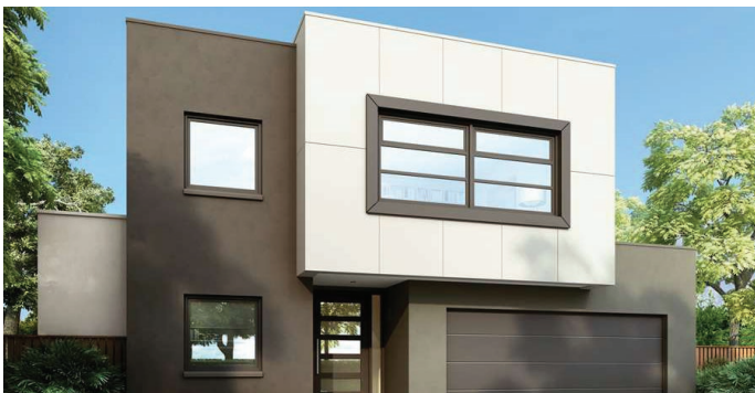
ARTICULATE upper floor walls. *image provided by Metricon.
