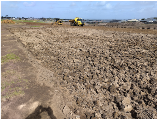
Fill area ripped prior to watering, compaction and placement of fill
