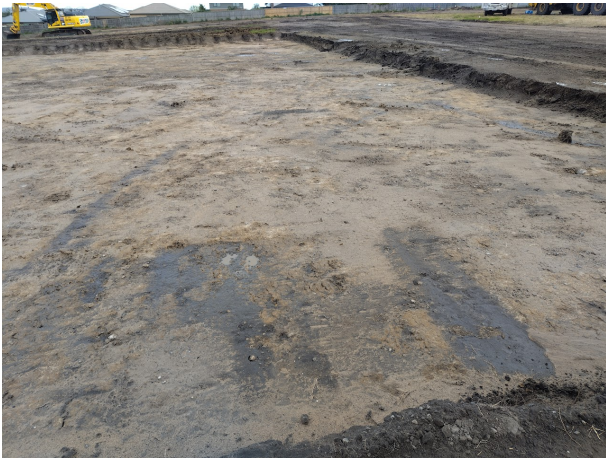
Site stripped and cleared of topsoil prior to placing fill
