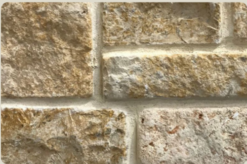
Stone cladding feature elements
