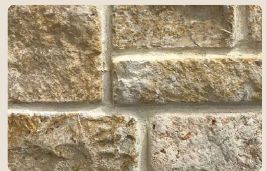
Stone cladding feature elements
