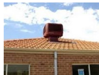
Standard unit in clear view of street. Not Acceptable
