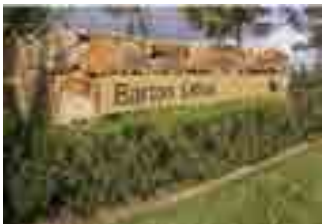
Street names in retaining walls
