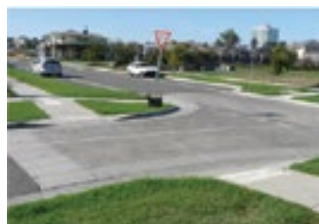
Charcoal coloured exposed aggregate concrete
