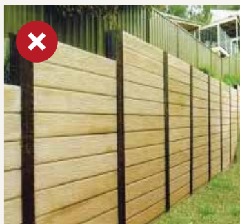
Not acceptable (where visible to public street).
