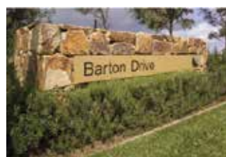
Street names in retaining walls
