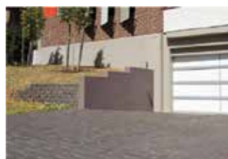
Porous paving, such as Boral Hydropave
