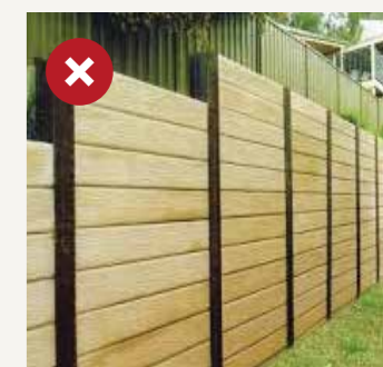
Not acceptable (where visible to public street).
