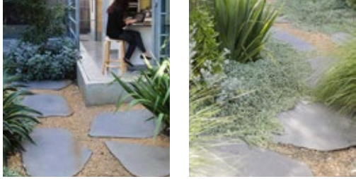
Concrete consolidated and compacted 'tuscan toppings'
