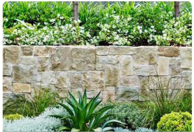
Terraced retaining wall. *image provided by Seed Landscapes.
