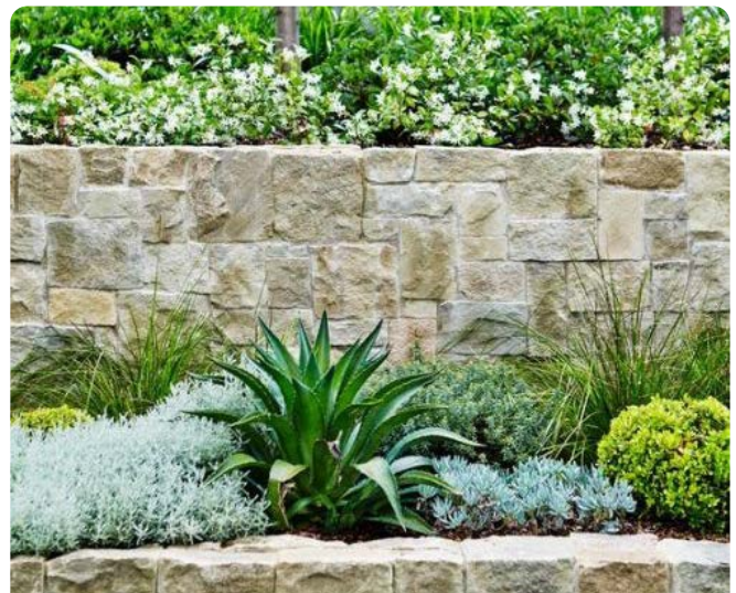
Terraced retaining wall. *image provided by Seed Landscapes.
