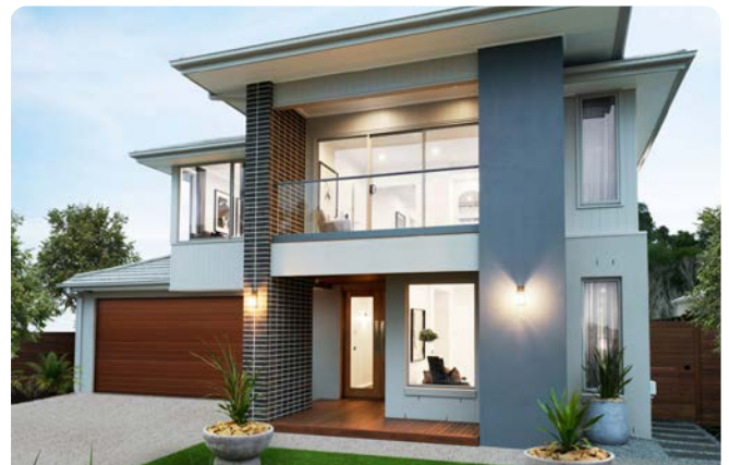
Limit face brick to smaller detail elements only. *image provided by Simonds.
