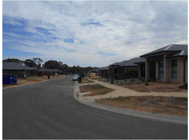
Figure 2. Low Threat development to the south of the site
