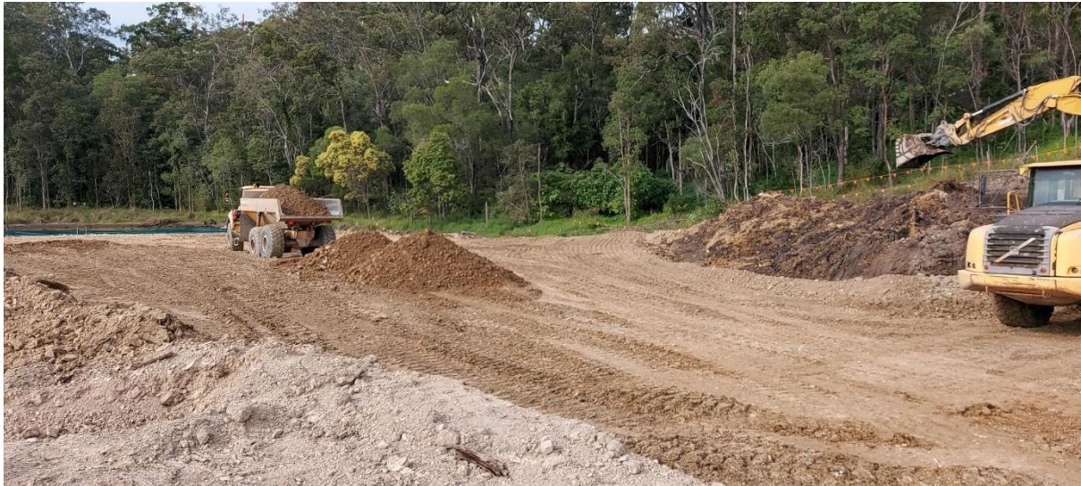
Image A – Construction of the bridging layer on Lots 15-17
