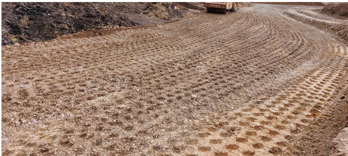
Image C – Placement of Fill over the bridging layer on Lot 14
