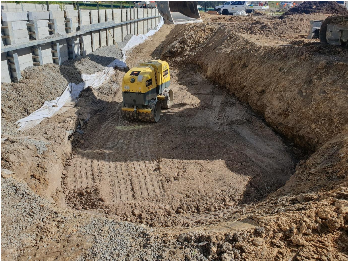
Image H – Compaction of the fill material behind the retaining wall on Lot 19
