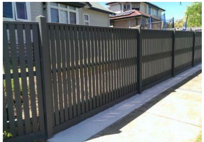
Example of 1.8m high capped 'hit and miss' paling with a minimum 25% transparency along Secondary Road Frontage.
