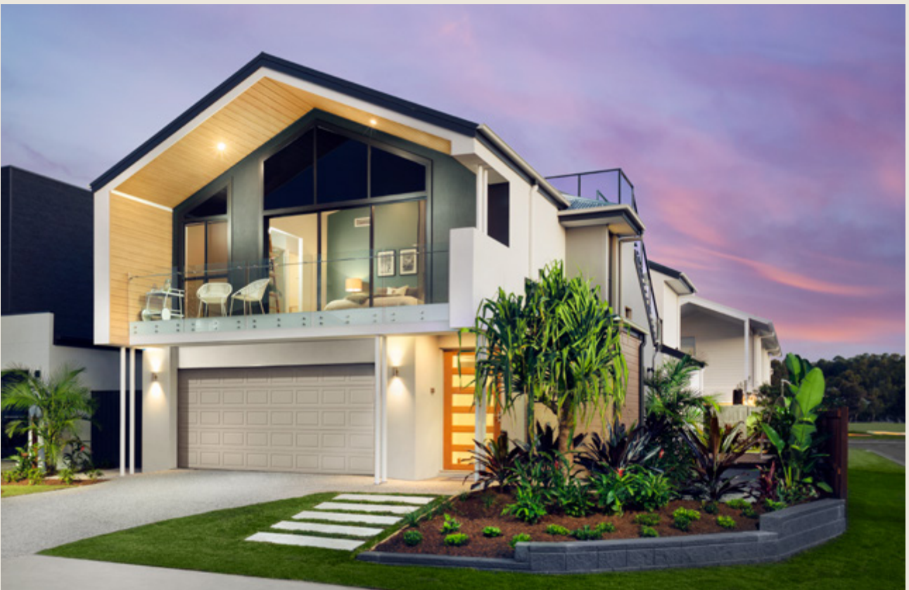
COURTESY OF OWNIT HOMES QLD – CORNER LANDSCAPING
