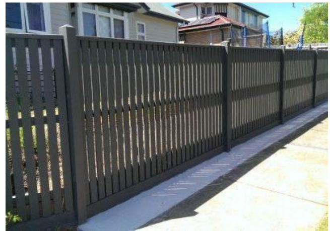
Example of 1.8m high capped 'hit and miss' palings with a minimum 25% transparency along Secondary Road Frontage.
