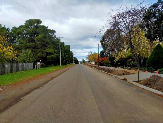
Figure 1. Main access via Ash Road, looking south from property
