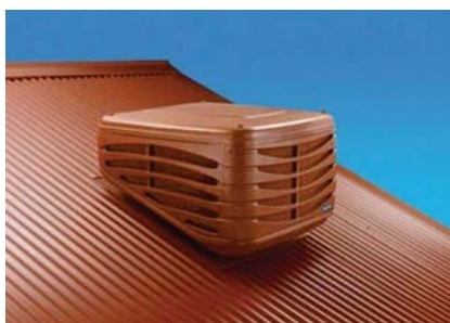
LOW PROFILE AND POSITIONED AT REAR ACCEPTABLE
