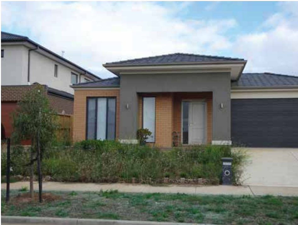
Above – Unacceptable – Lack of Maintenance
