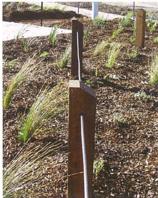
1 TIMBER POST AND CABLE VEHICLE EXCLUSION FENCING (SUPPLIED BY CITY OF WHITTLESEA)
