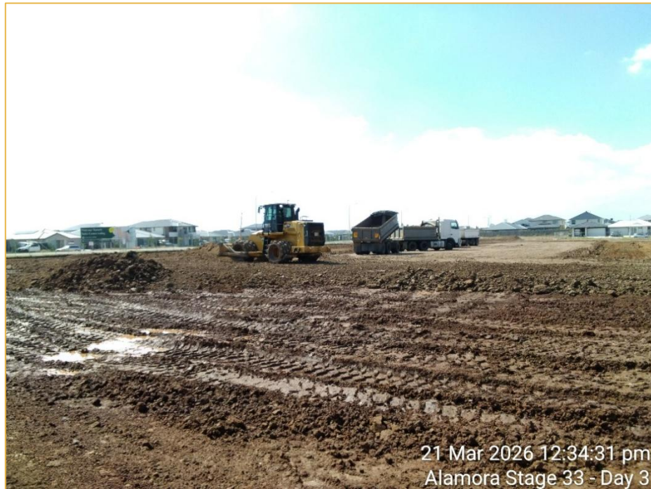
Figure 5: Fill Compaction with 815 Compactor (Source: CTGM)
