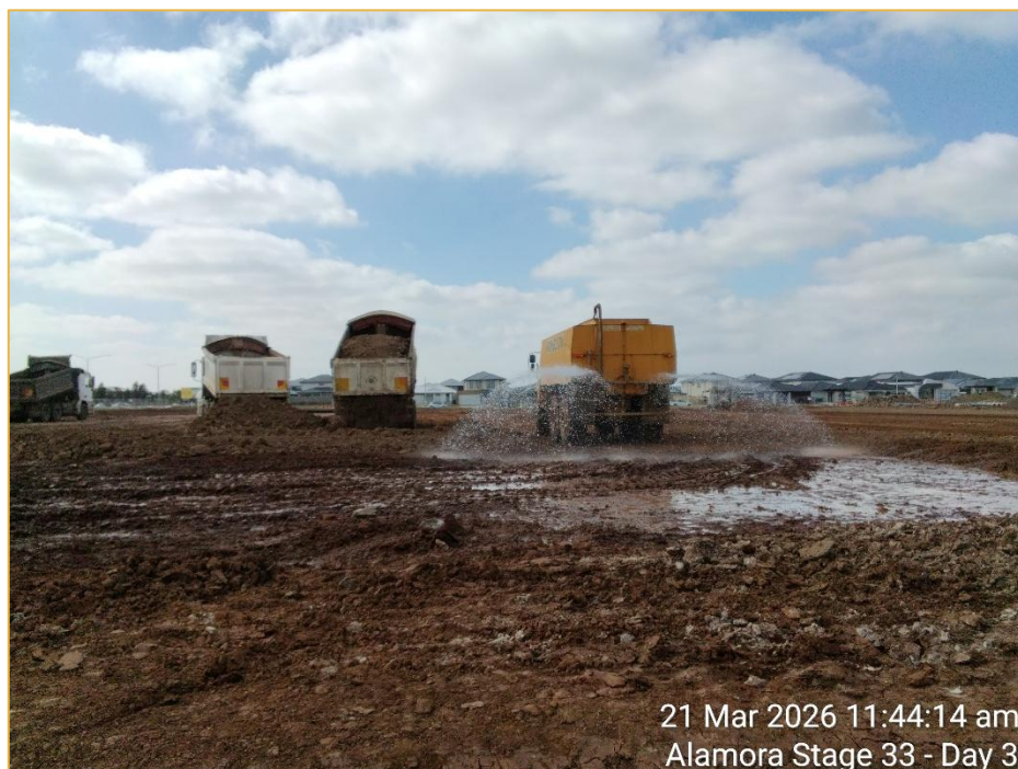
Figure 4: Fill Placement – Carting Fill to Site and Moisture Conditioning (Source: CTGM)
