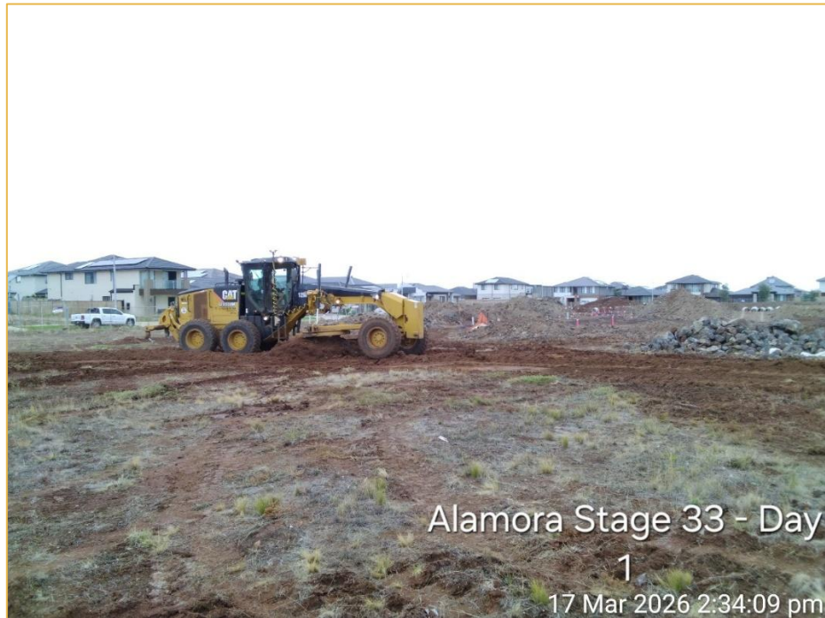
Figure 2: Subgrade Preparation – Topsoil Stripping (Source: CTGM)
