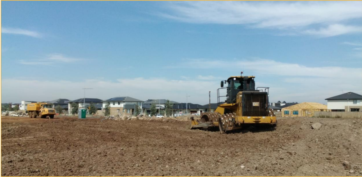
Figure 3: Fill Compaction (Source: C&T)
