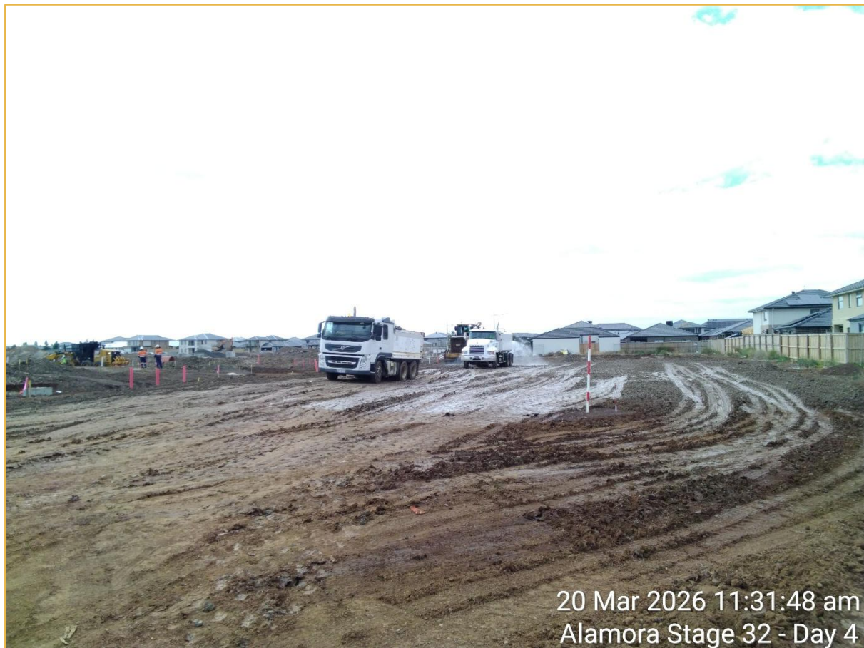
Figure 2: Moisture Conditioning During Fill Placement (Source: C&T)
