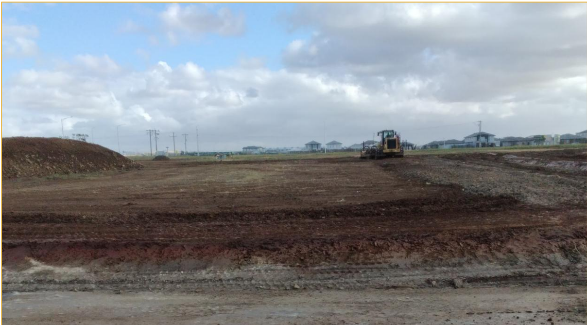
Figure 1: Subgrade Preparation (Source: C&T)
