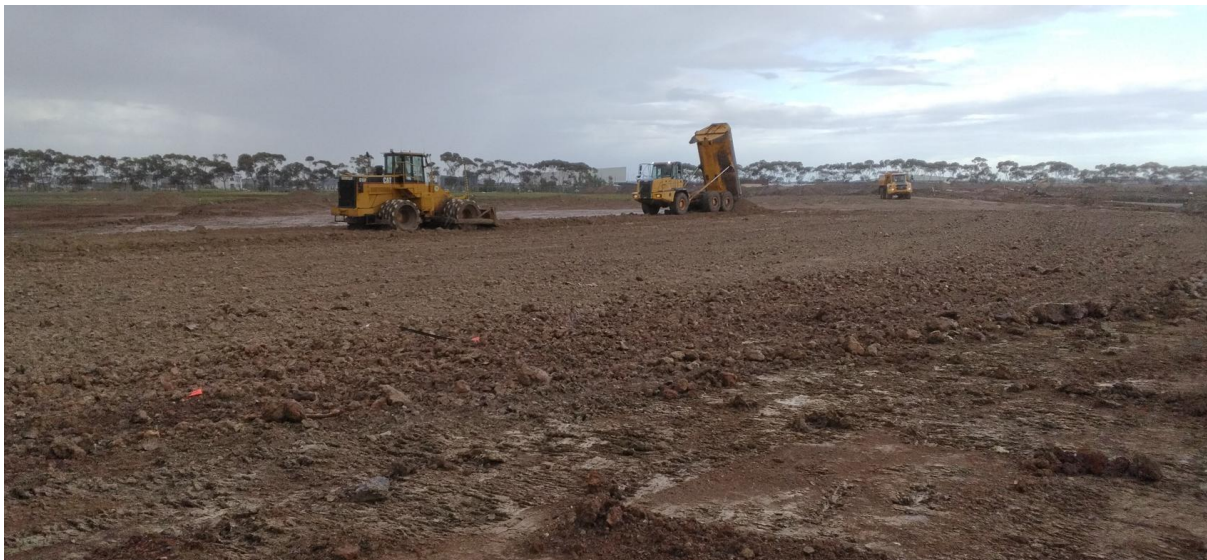
Figure 3: Fill Spread and Compacted (Source: C&T)
