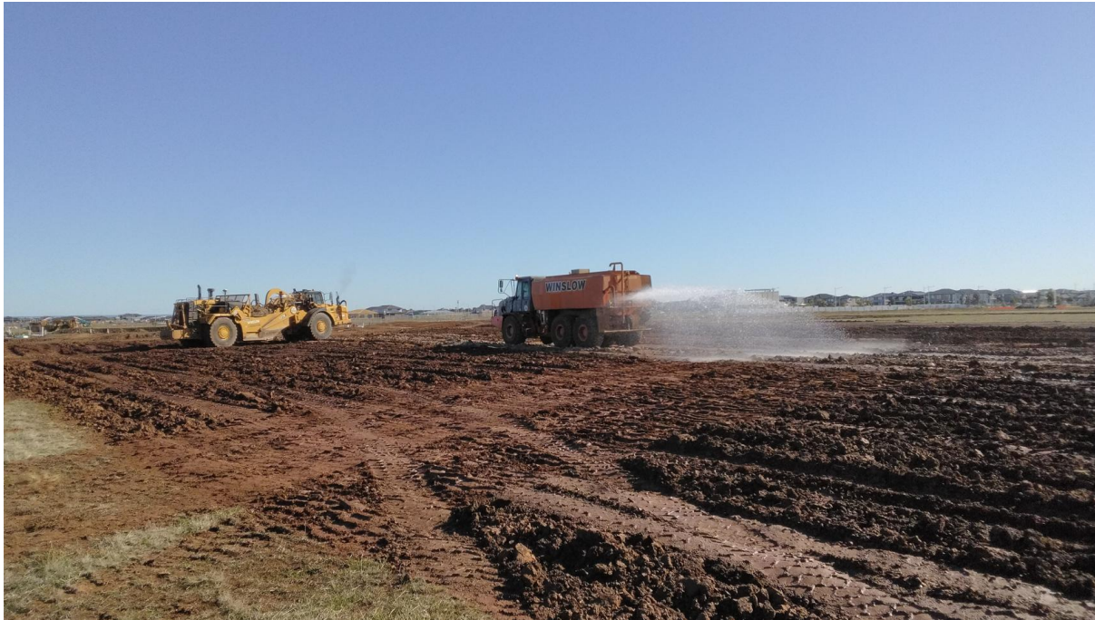
Figure 2: Fill Being Moisture Conditioned During Placement (Source: C&T)
