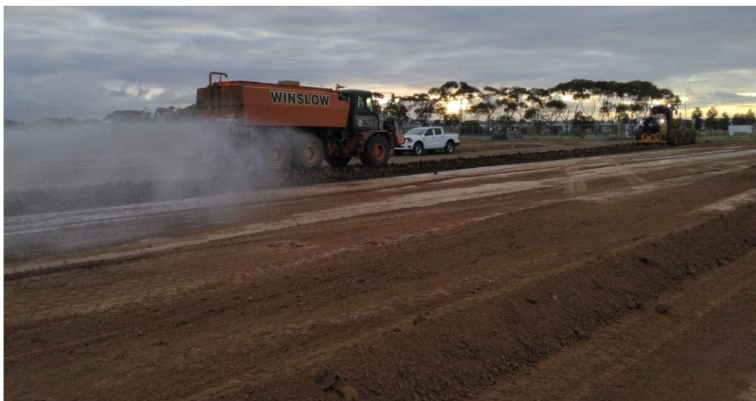
Figure 1: Moisture Conditioning of the Subgrade (Source: C&T)
