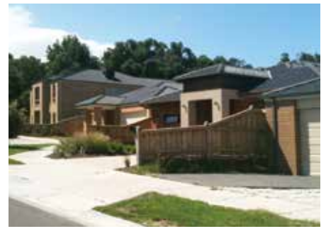
INCORRECT FENCE STYLE
