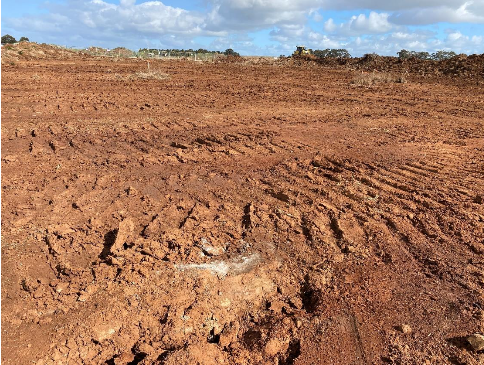
Site Photo 1: Showing the stripped ground surface
