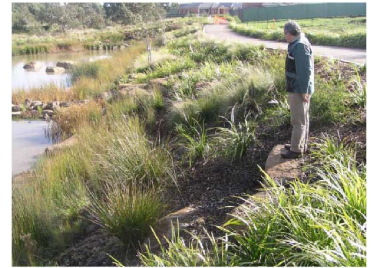
TYPICAL ROCK STEPPED EMBANKMENT
