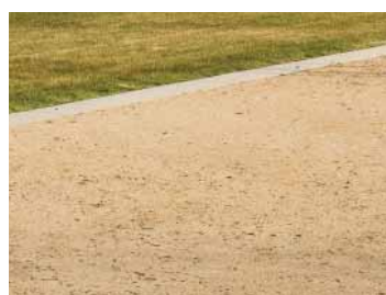
Tuscan Toppings Figure B25 - Parkland Paving
