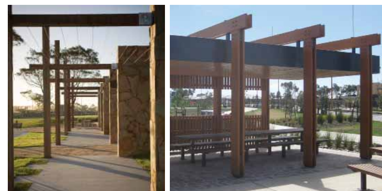
Figure B37 - Parkland Furniture Elements - refined stone, steel and composite timber structures
