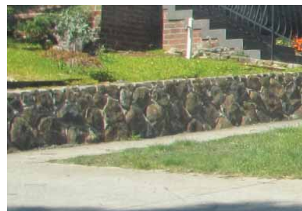
Figure B34 - Bluestone retaining walls* on Loop Connector street (consistent for full length.)
