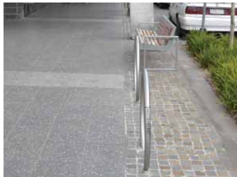
Figure B23 - Precast and stone highlight paving* in retail core of Town Centre
