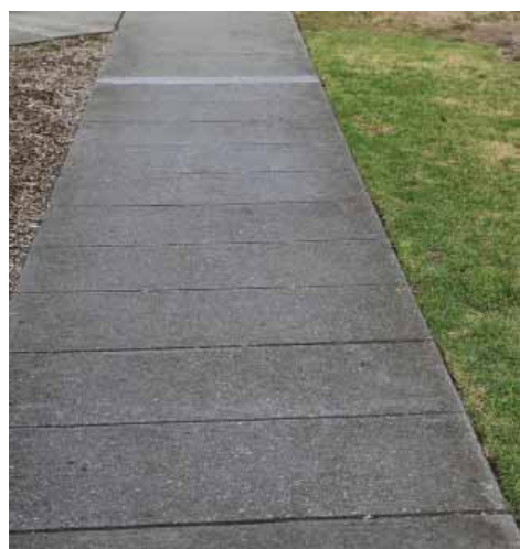
Figure B24 - Charcoal coloured concrete paving in residential streets of Town Centre*
