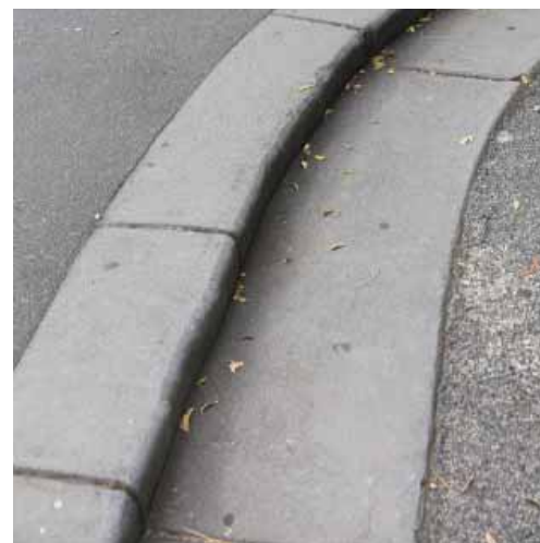
Figure B28 - Special profile charcoal coloured kerb and channel in Town Centre*
