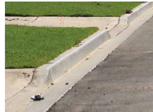
Figure B26 - Plain concrete kerb and channel*
