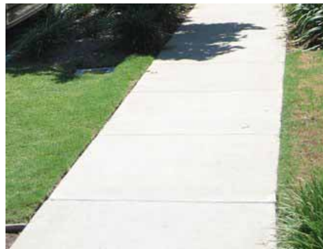
Figure B22 - Plain concrete* scored at 1500
