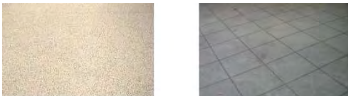
Figure 13: Examples of approved driveway finished.
