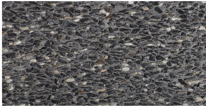
Example of exposed aggregate concrete.
