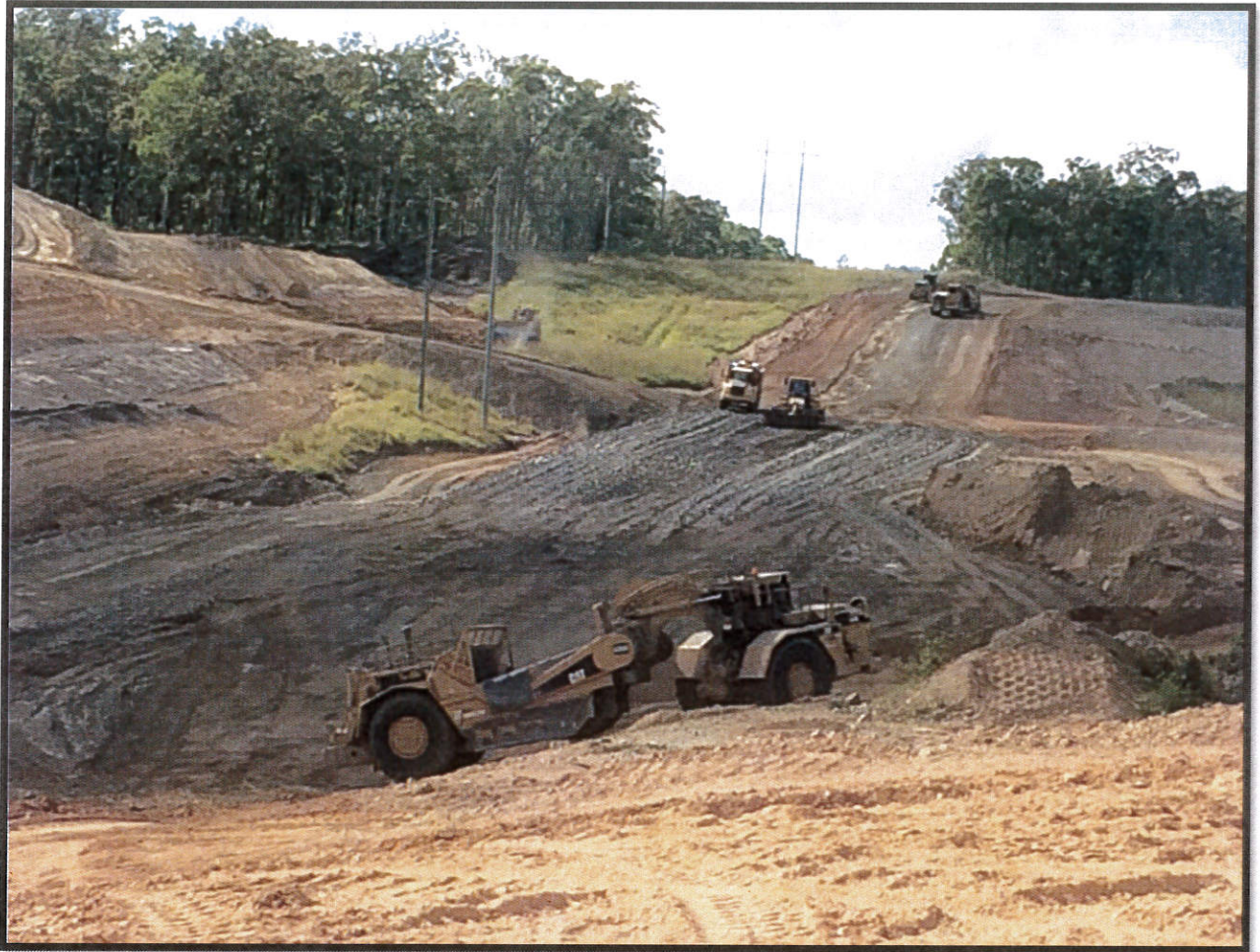
Picture 3: Site Earthworks Filling Operations
