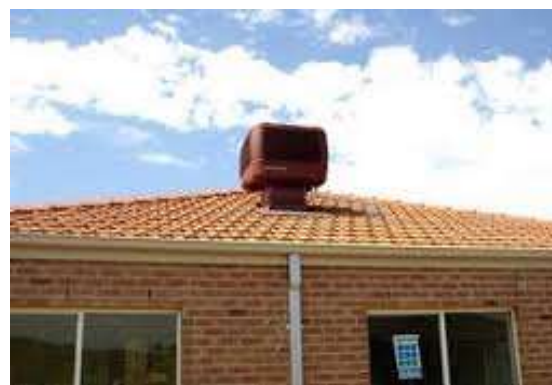
Standard unit in clear view of street Not acceptable
