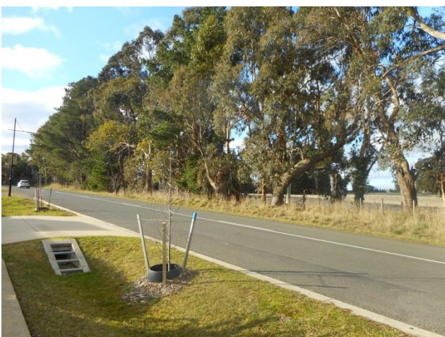
Figure 5. Low Threat areas along Old Lancefield Road
